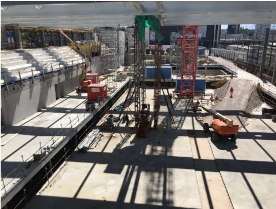
The future 50m-pool in the Malley complex
